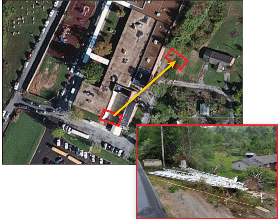
Figure B3-15. Flying debris hazard: an EF1 tornado blew a school gymnasium's steel truss and steel deck roof assembly approximately 230 feet (Cleveland, TN, 2011)
