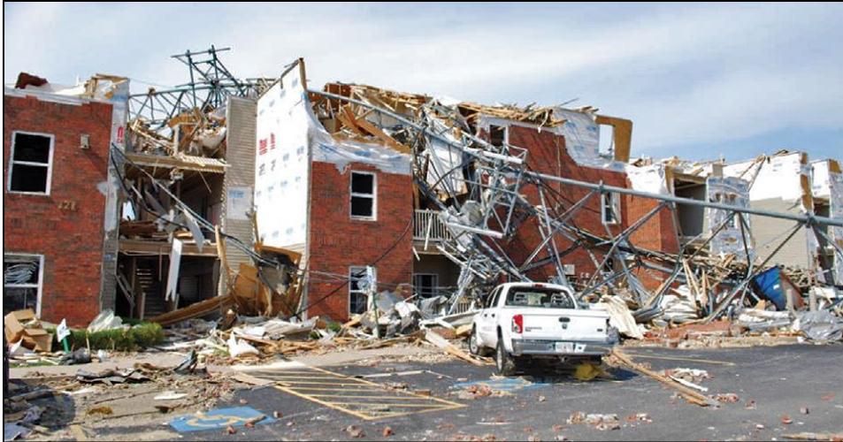
Figure B3-12. Lay down hazard: failure of a large communications tower onto a building (Joplin, MO, 2011 tornado) (SOURCE: FEMA P-908, RECOVERY ADVISORY 5)
