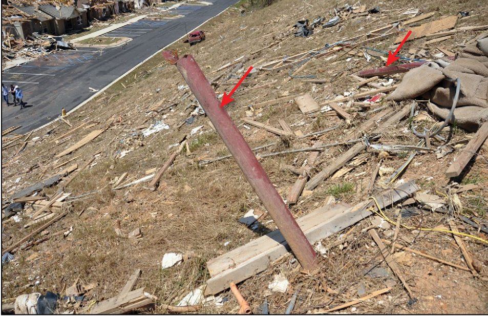
Figure B8-19. Steel porch column debris from an apartment complex where columns that were 7 feet 9 inches long and 4¼ inches in diameter (see red arrows) had a significant upward trajectory and flew approximately 230 feet (Tuscaloosa, AL, 2011 tornado)
